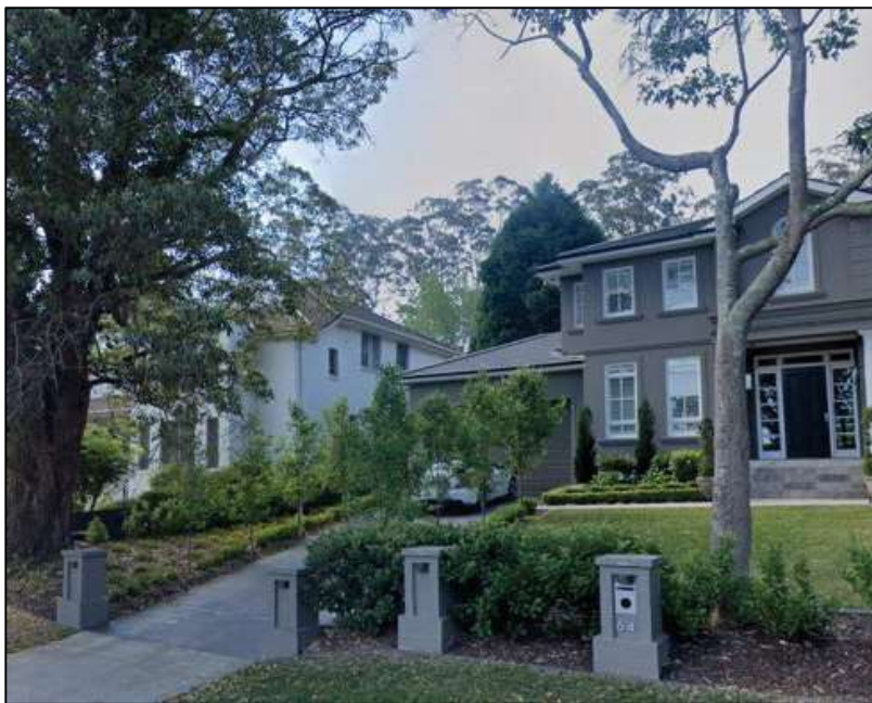
Figure 13: Nos. 62 and 64 Billyard Avenue adjacent to the southeast of the subject site.
